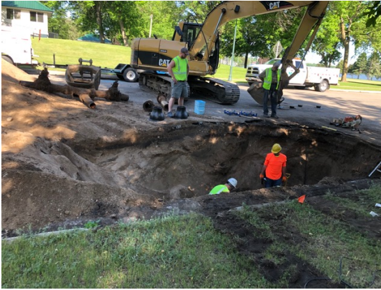
Public Works Staff working to replace leaking valves installed in 1922.
