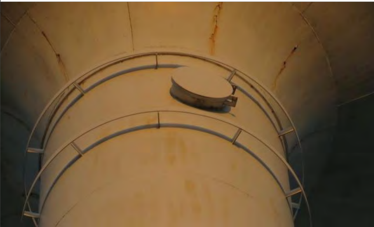
Photograph #: 8 Date: September 29, 2021 & August 24, 2022 ~ 300,000 Gallon Elevated Storage Tank ~ Annandale, MN Subject: View of Painter's ring and hatch
