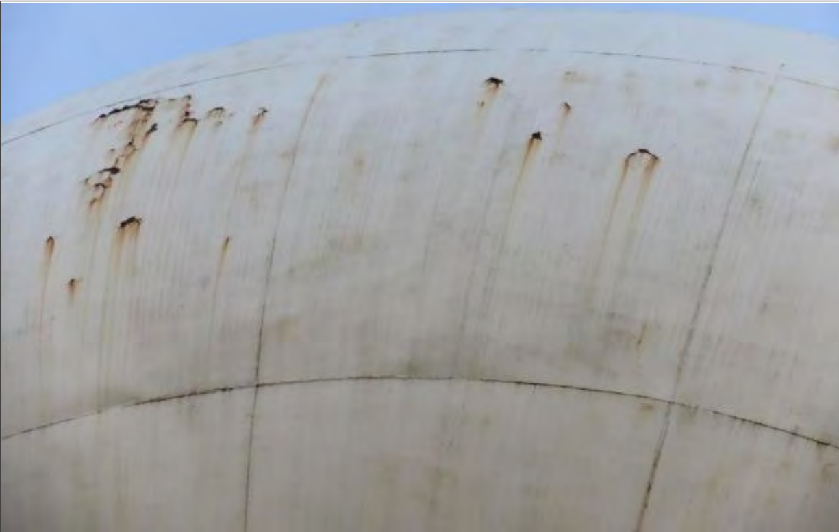
Photograph #: 7 Date: September 29, 2021 & August 24, 2022 ~ 300,000 Gallon Elevated Storage Tank ~ Annandale, MN Subject: View of tank shell (Note: Corrosion)
